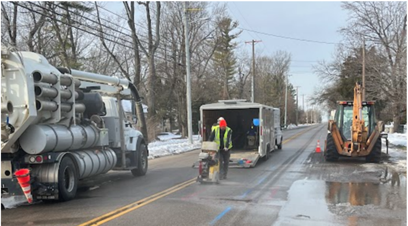
Recent water main break repairs.
